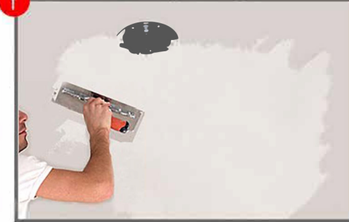
Step E- With Plaster receiver tightly secure against GWB, add GWB screws to further secure plaster receiver. Step F- Apply tape and joint compound (dry). Plaster over ceiling and receiver.
