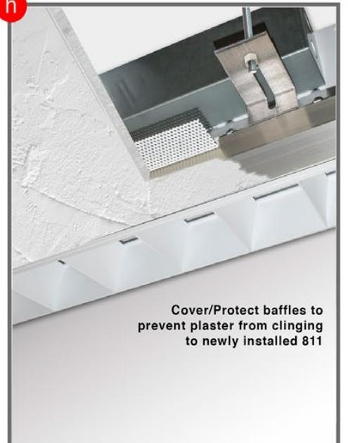
**Step H-** Plaster over screed edge of plaster frame. Finish GWB install and plaster coating.
