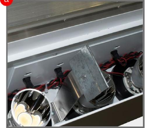
**Detail-** Closeup showing inverted v- shape metal bracket. Applying pressure on both sides of bracket will release baffle from housing
