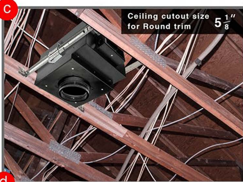
Exposed Ceiling Joists. Connect all wiring for housing before ceiling installation.
