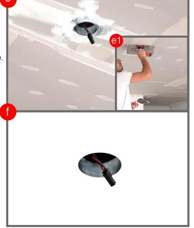
**Step E-** Plaster receiver flange. **Step F-** Finish Ceiling. Assure no paint or other debris impede electrical connection or interfere with fixture attachment.
