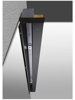
Step 1- Add blocking to support mounting screws. Cut ceiling to fit housing. Fit housing into corner and anchor with mounting screws into top plaster flange and side wall flange.
