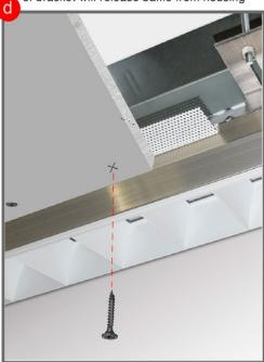
Step D- GWB goes around plaster frame and housing, use factory edge against plaster frame. Fasten frame to GWB with sheetrock screws that anchor into perforated metal tabs attached to Ultrim frame.
