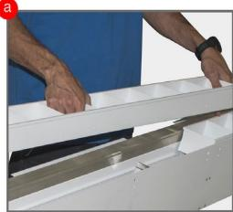
Step A- Remove baffles from housing before anchoring unit to wall. Baffles must be removed to access holes for anchoring housing to wall.
