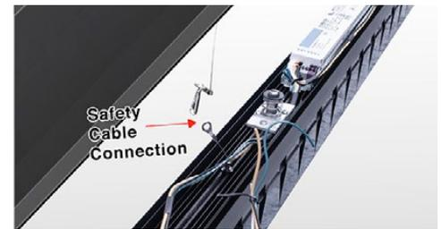
Step 3- Connect power to leads from driver to complete electrical connections. Secure safety cable connection.
