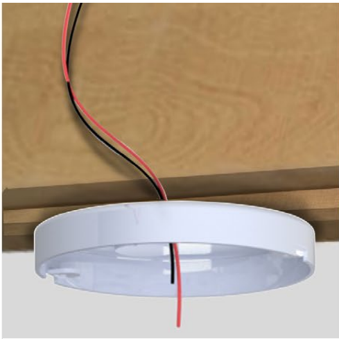
Step 1- Attach 4" diameter pancake box to structure. Pull wires from remotely located driver through knock outs in pancake box.
